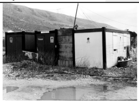
These are refugee shelters in a camp near Mostar. They are 20 foot shipping containers modified with windows, a door and an electrical connection. We met
